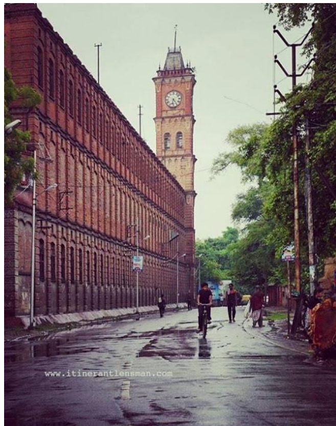
Figure 2- Building structure of Lal Imli
