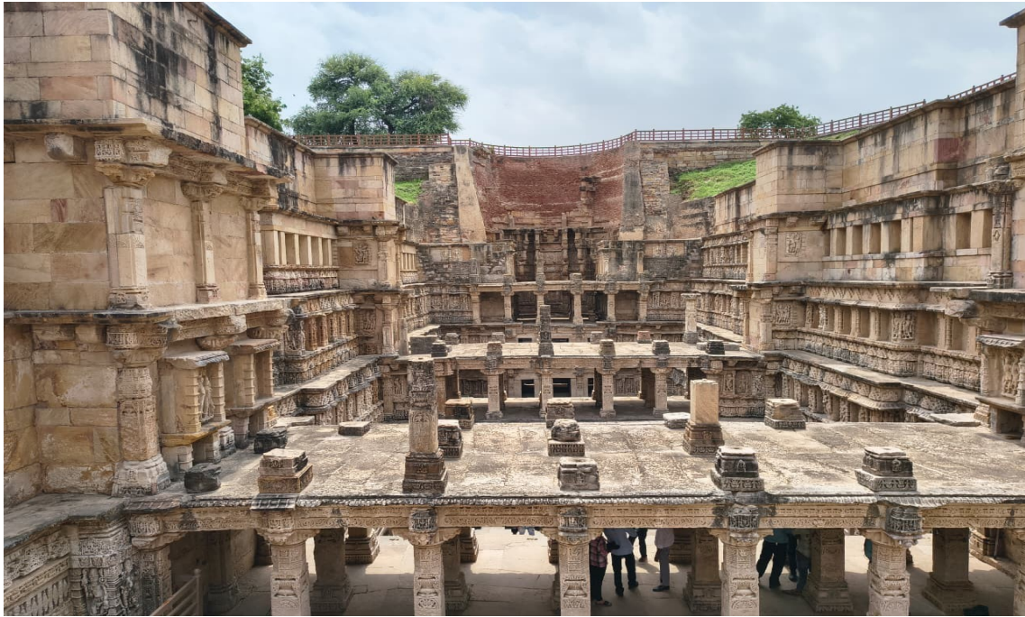
Figure 7: General view of the stepped corridor and pavilion tiers
