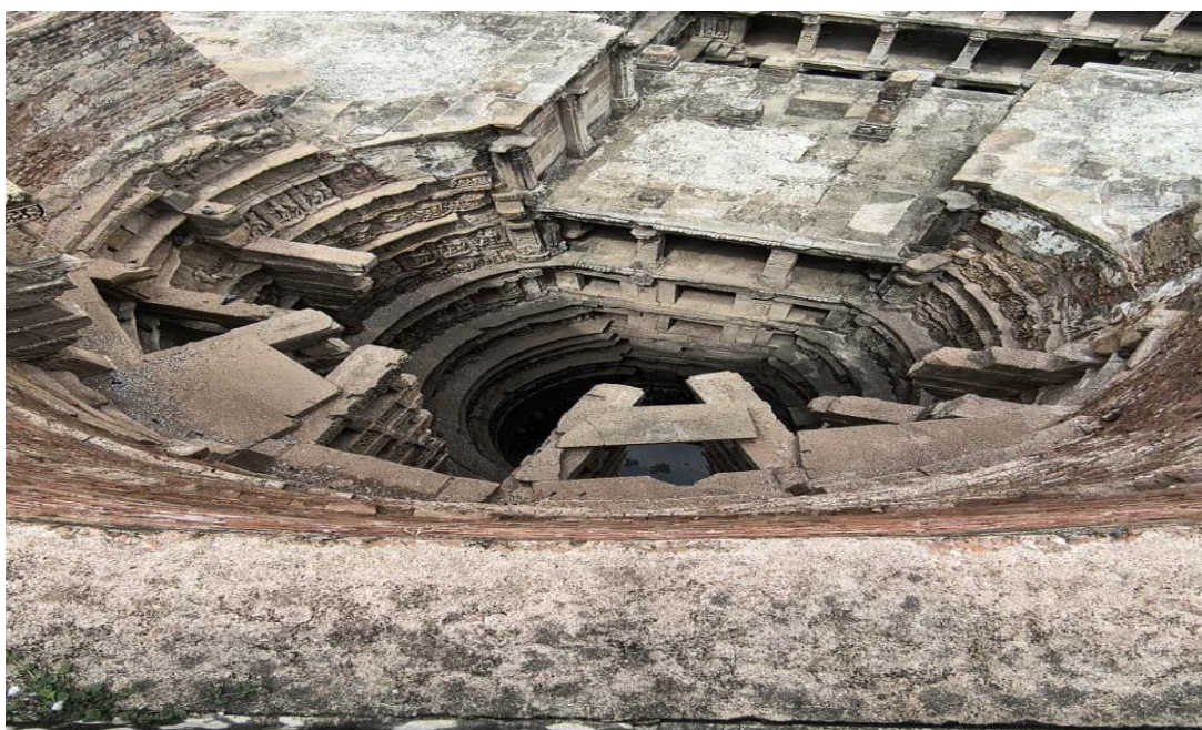
Figure 9: The well shaft viewed from above
