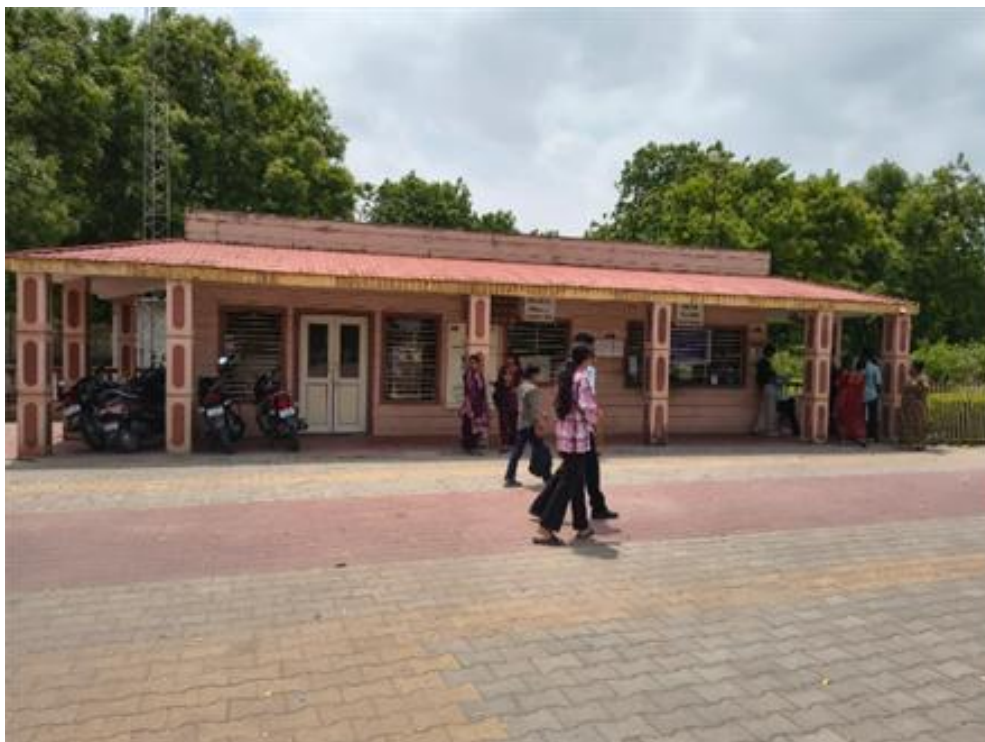
Figure 13: Ticket office and visitor facility building
